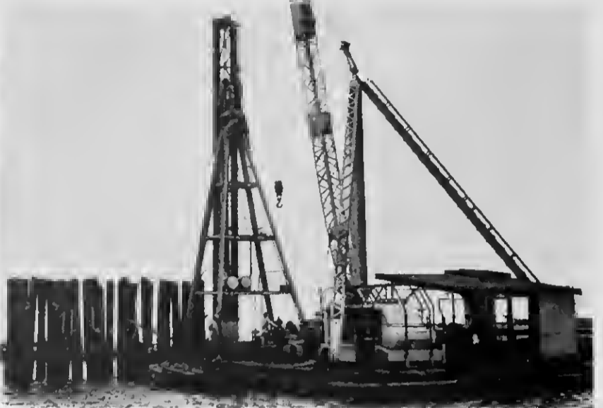
A NEW dolphin is going up in the harbor near the entrance, to be put in use sometime next month. The idea is to relieve dock congestion by berthing ships on the dolphin if they have minor repairs or are taking on bunkers.
